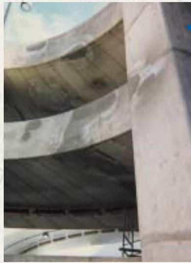
**SHOTCRETE** — AR-CRACKNON is used in shotcrete applications for repair of structural concrete because it resists drying shrinkage cracks and is easy to handle, mix, pump, and spray. Finishing is easy since the fibers lie down smooth within the concrete (no hairiness) and are not visible on the surface. High fiber contents are possible so crack-free shotcrete can be produced.
